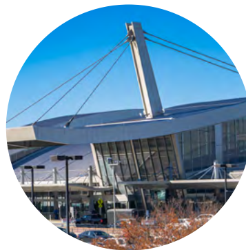
Terminal 2 Landside Expansion
